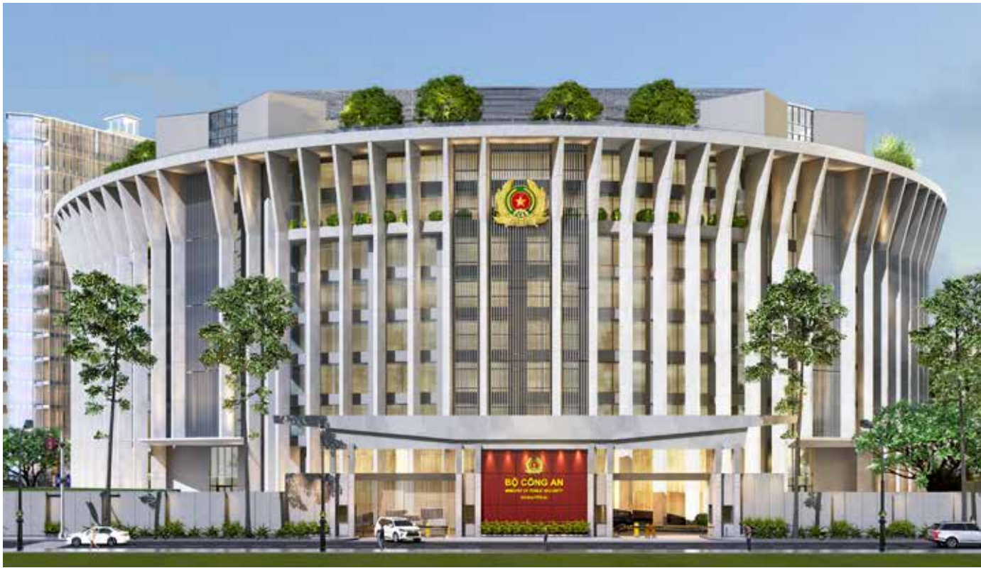
TS01.1-12 (MINISTRY OF PUBLIC SECURITY HEADQUARTERS) Location: 44 Yet Kieu, Hanoi Client: TS01.1-12 Project Management Board Implementation period: 2024 Services provided: Construction supervision consultancy
