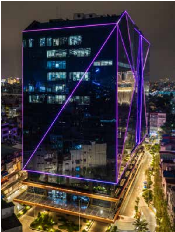
OFFICE BUILDING OF VIETNAM NATIONAL PETROLEUM GROUP
