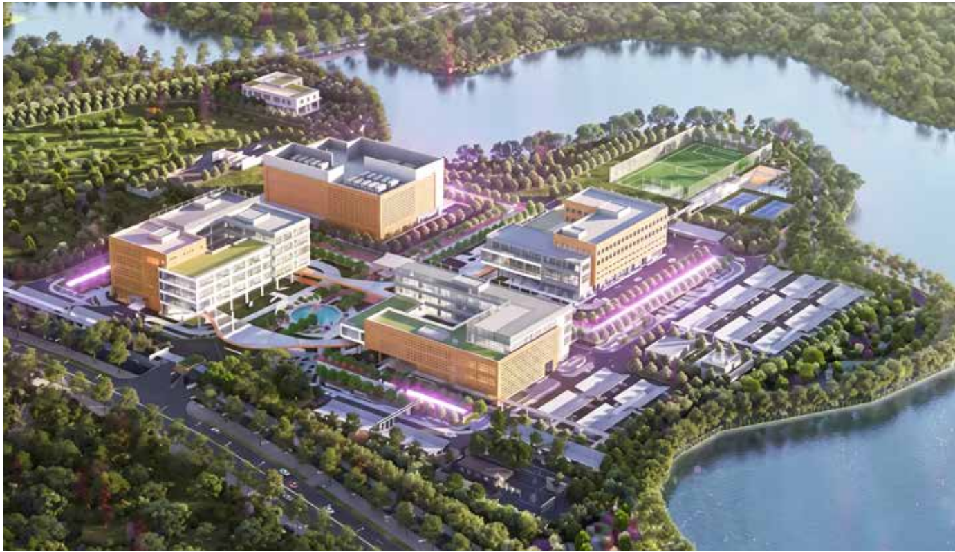
NATIONAL DATA CENTER NO. 1 Location: Hanoi Client: National Data Center Implementation period: 2025 Services provided: Supervision of construction and equipment installation
