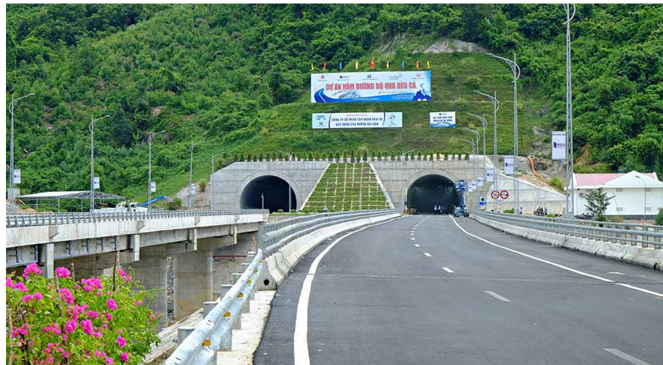
TUNNEL CONSTRUCTION PROJECT THROUGH DEO CA PASS, NATIONAL HIGHWAY 1, PHU YEN AND KHANH HOA PROVINCES
